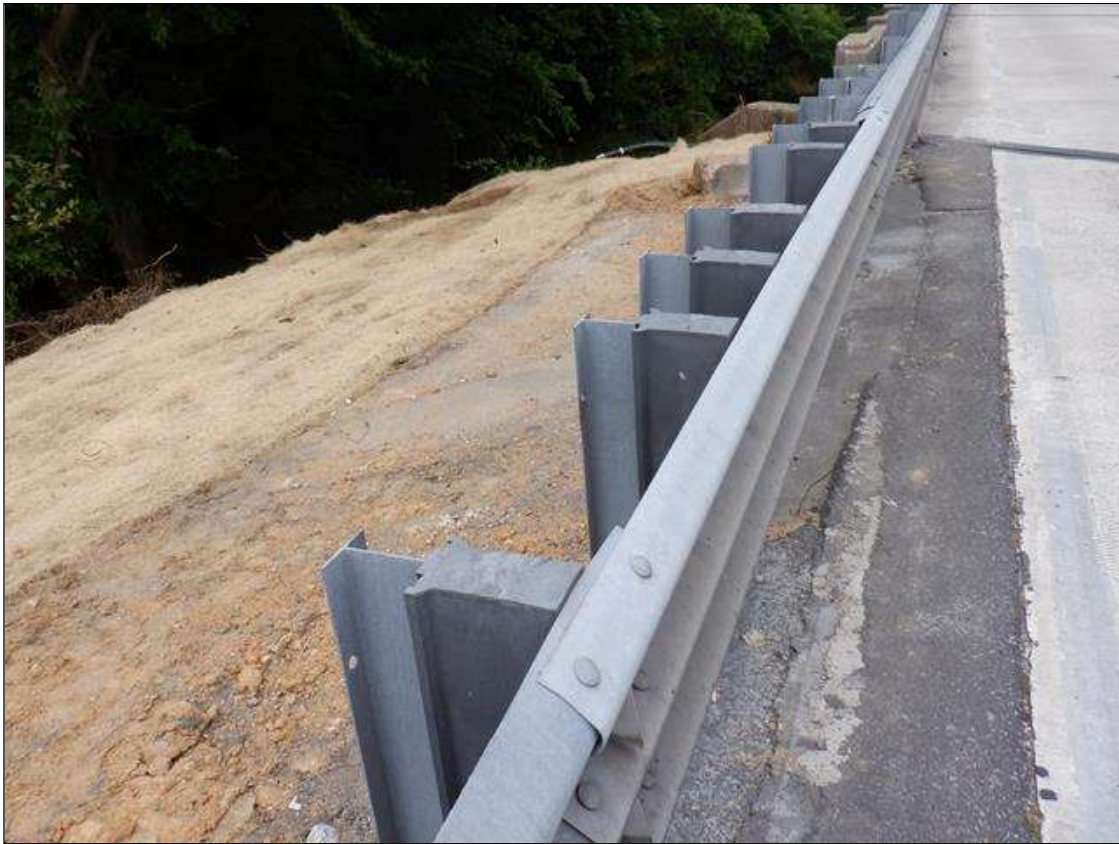
SOUTHWEST GUARDRAIL TRANSITION
