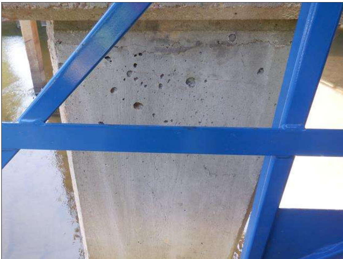
Bent 4 Pile 1: 5 FEET LONG X 0.02 INCH WIDE VERTICAL CRACK, SOUTH FACE BEGINNING AT CAP.
