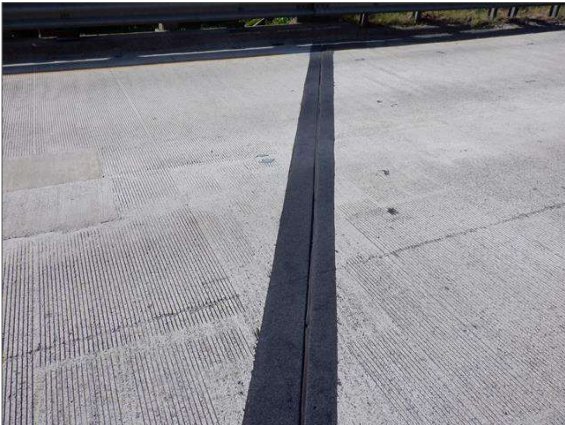
END BENT 1 JOINT
