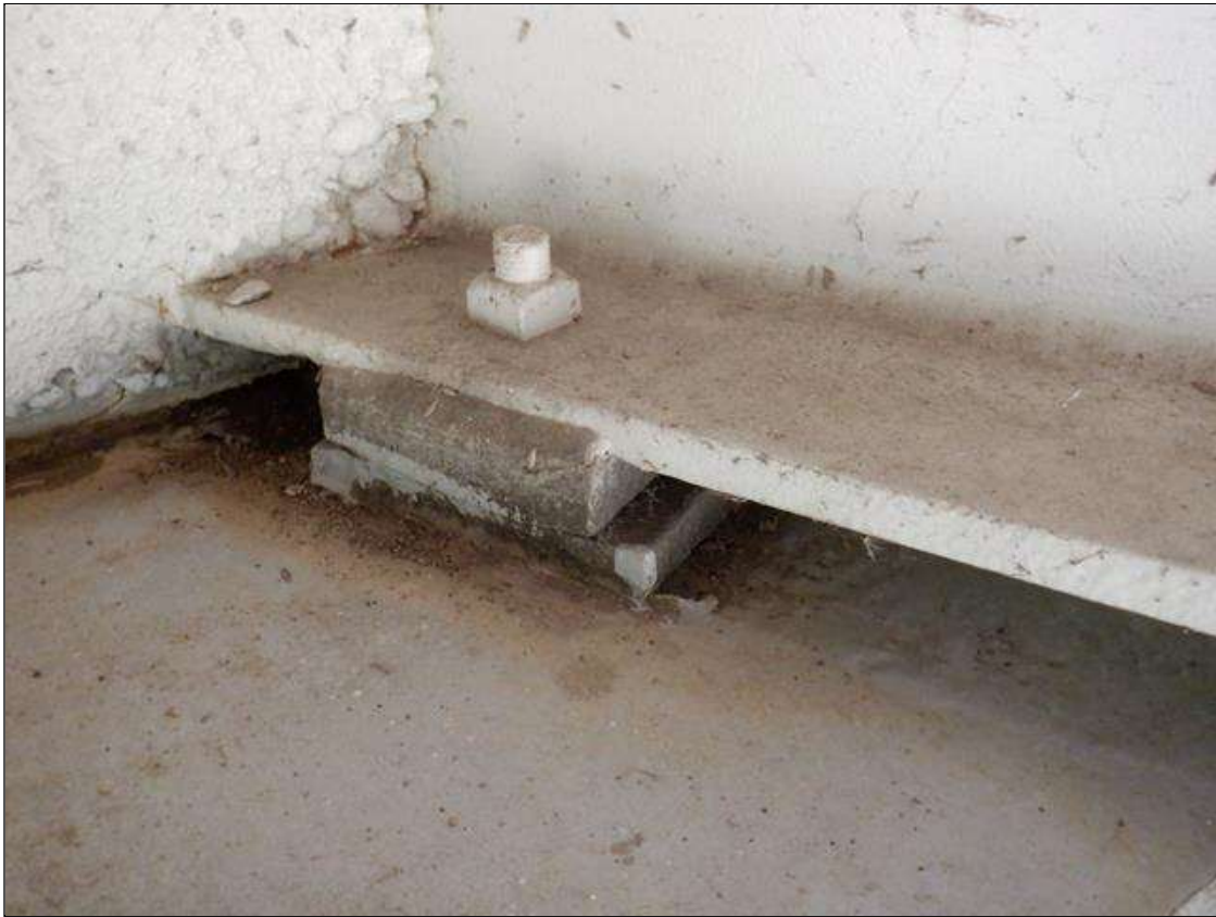
SPAN 8 BEAM 2 FAR BEARING
