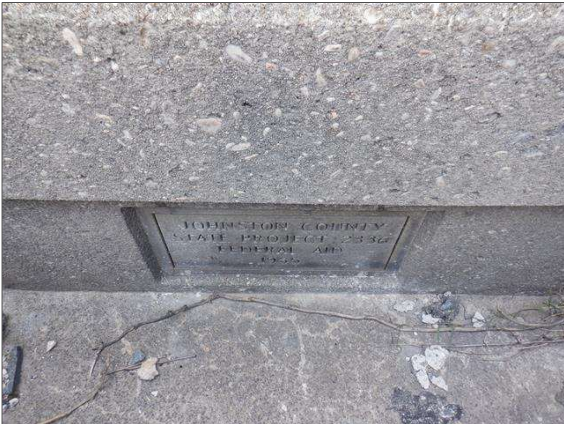
NORTHWEST CORNER BRIDGE PLAQUE
