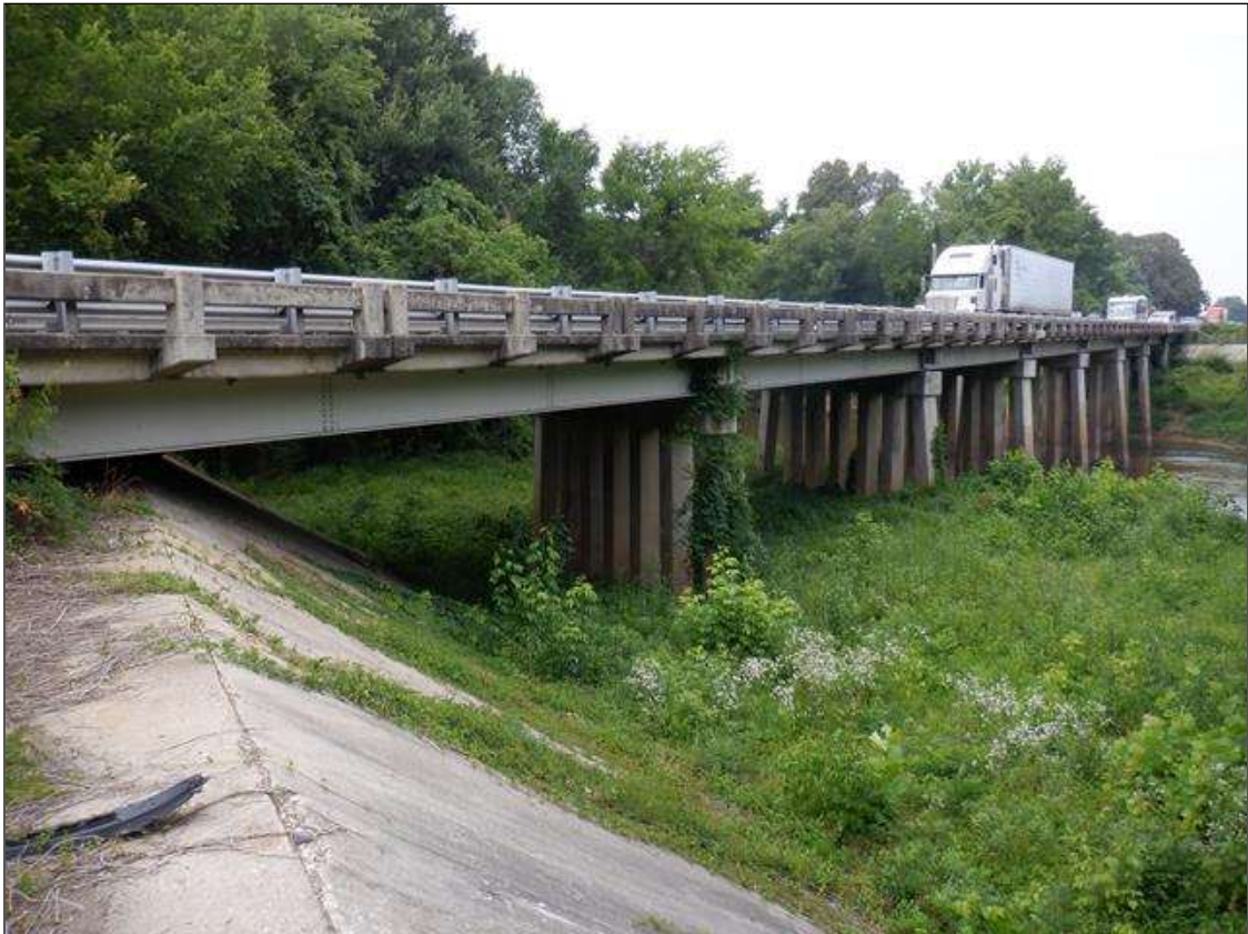
DOWNSTREAM STRUCTURE PROFILE
