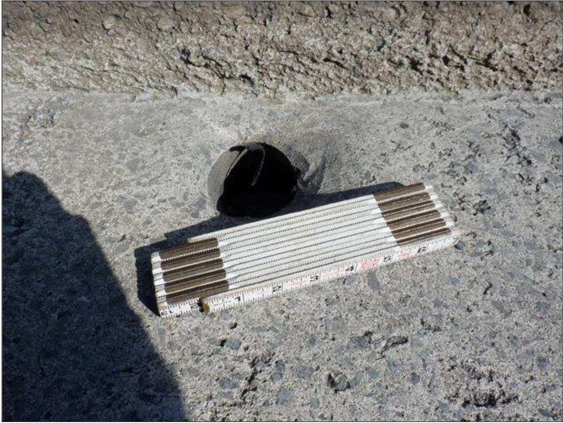
SPAN 7 ALONG LEFT BRIDGE RAIL 3 INCHES DIAMETER SCUPPER
