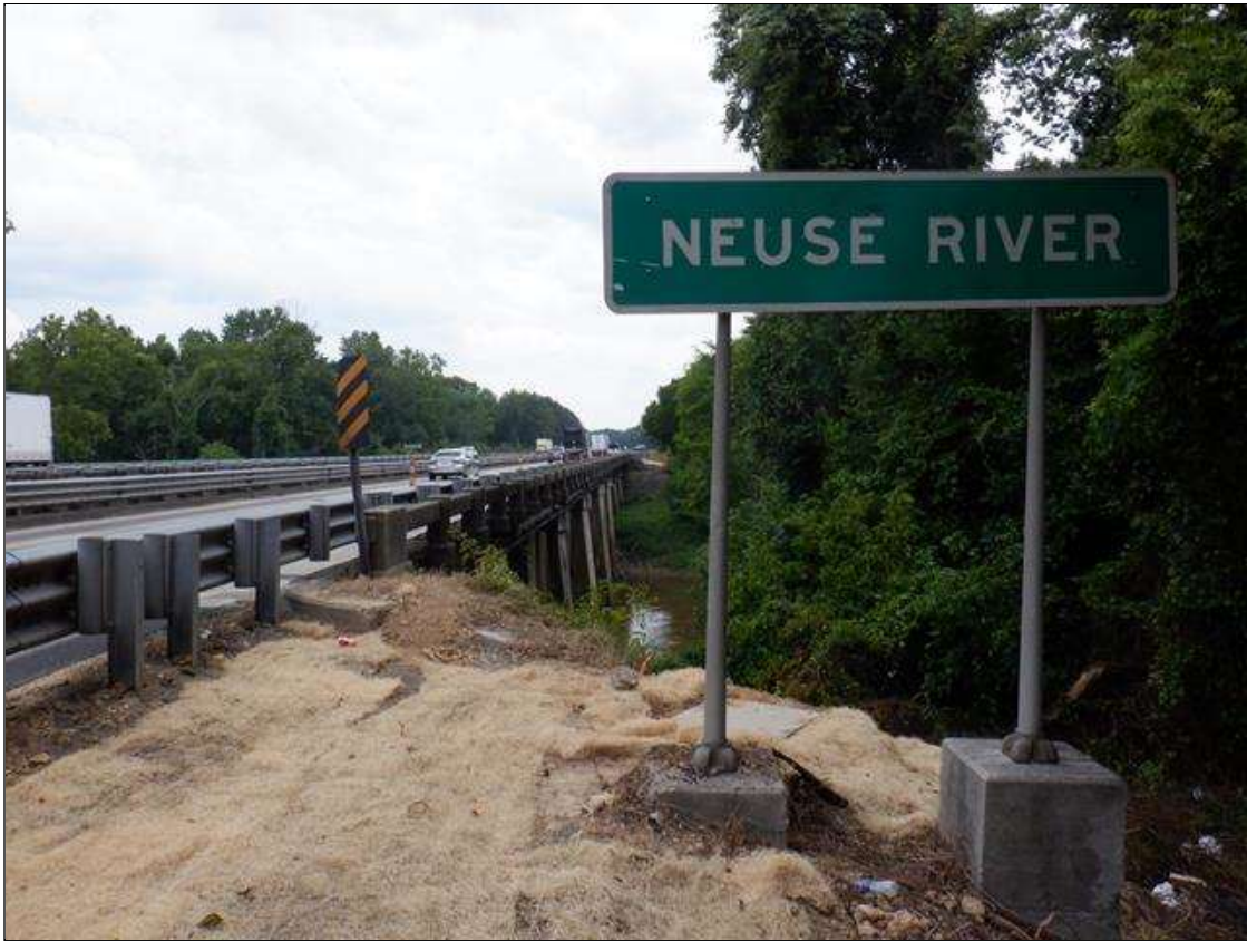
NEUSE RIVER SIGN AT NORTHWEST.
