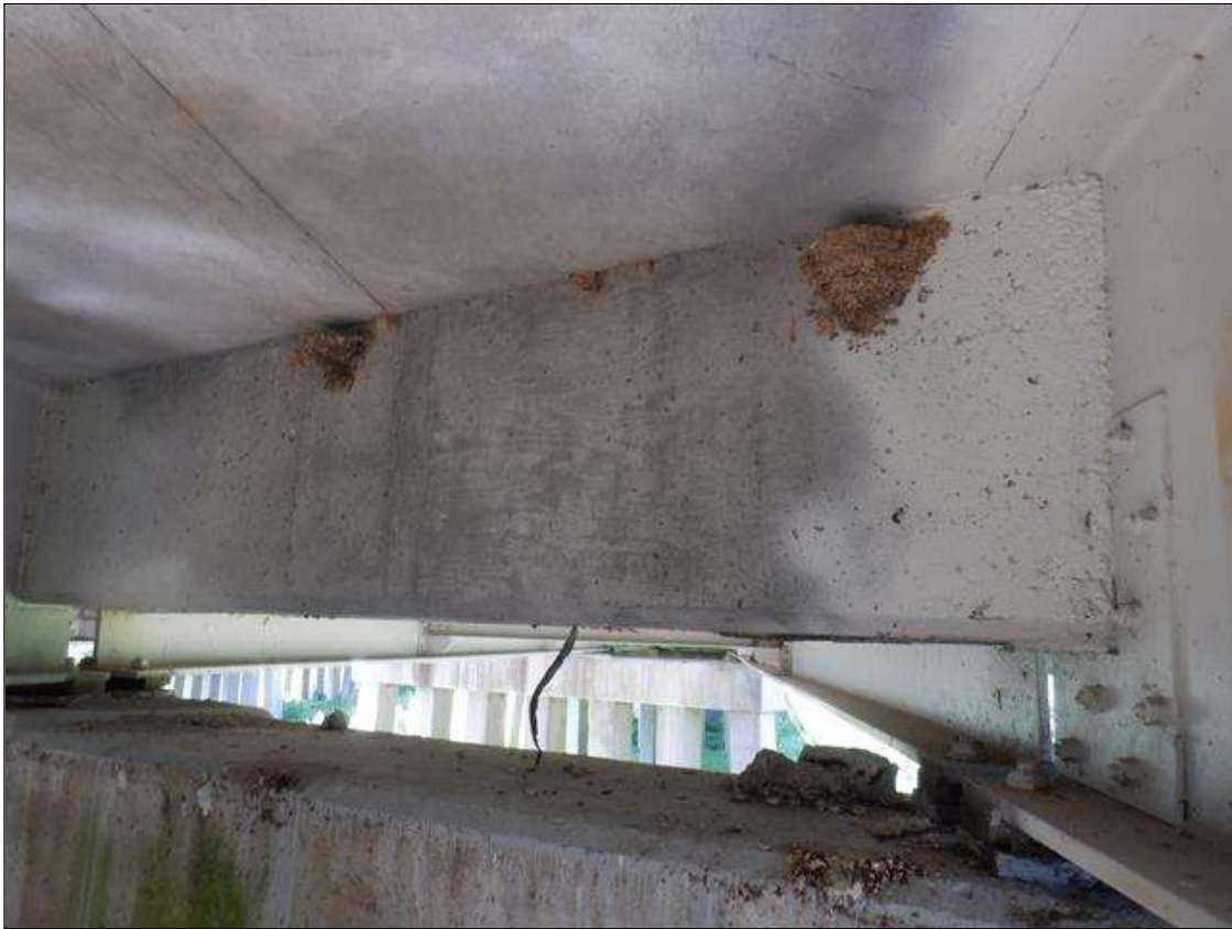
SPAN 5 BAY 1 NEAR END DIAPHRAGM
