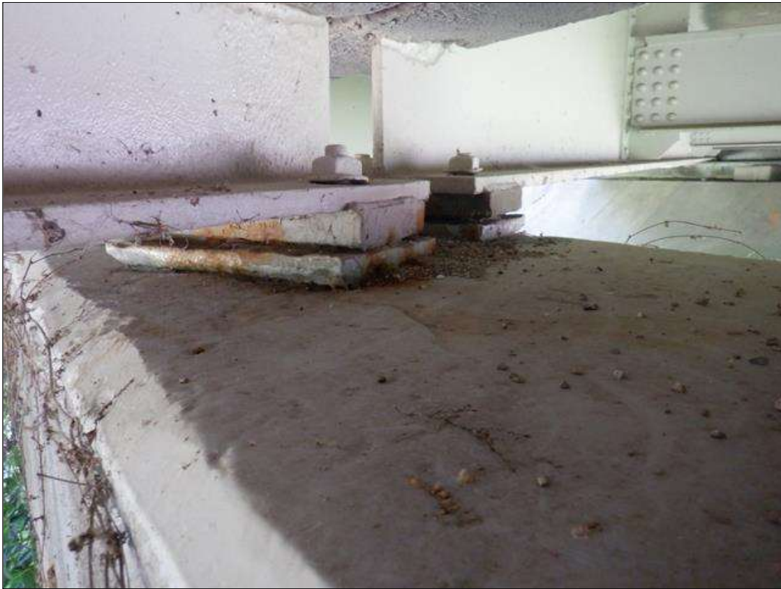
BENT 7 BEAM 2 BEARINGS
