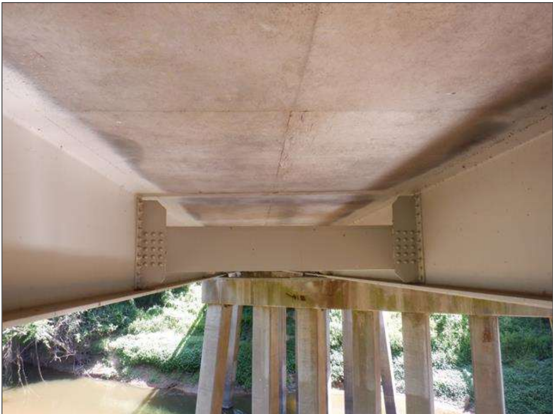
SPAN 5 BAY 1 INTERMEDIATE DIAPHRAGM
