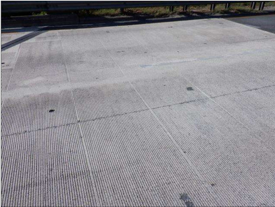
SOUTH APPROACH SLAB
